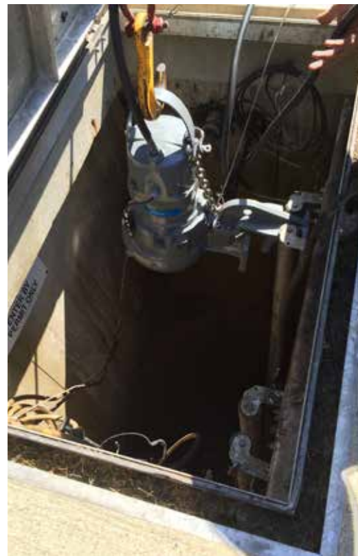
New Concertor™ pump being lowered into the wet well.
