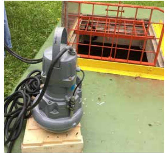
Concertor waiting to to be installed in the Crystal Lake pump station
