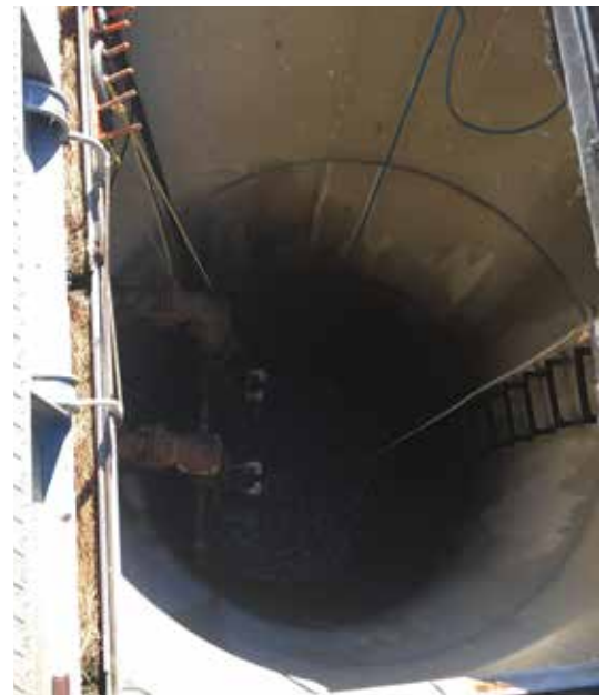
Down in the sump
